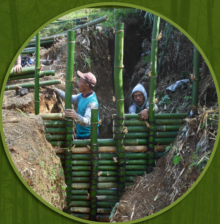
Bamboo gully plugs to prevent erosion and sedimentation, and to control gully development. Photo credit: WMTC
